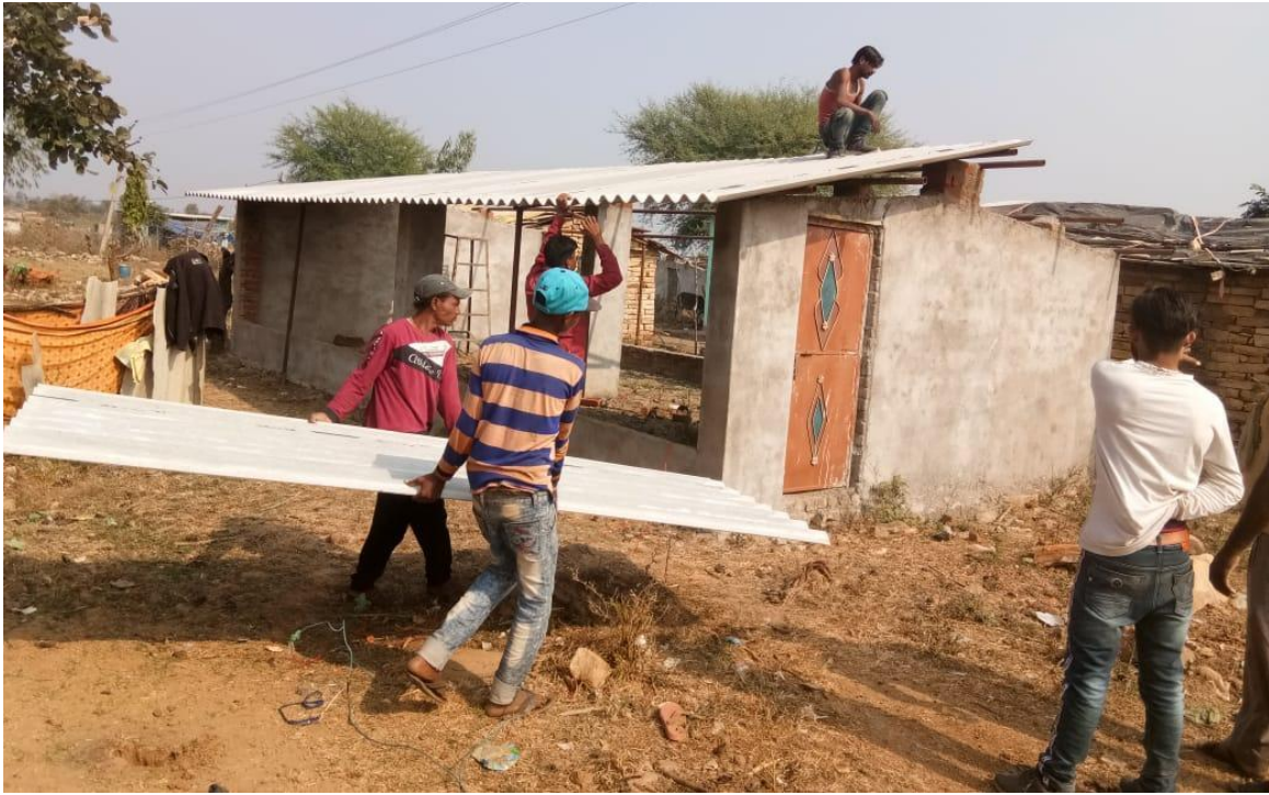
Figure 2 Construnction of poultry farming shed underway
